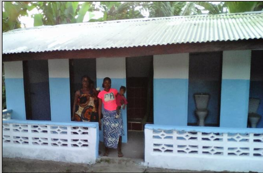
5-room bath and toilet house, Sarpawean Village, Margibi County, Liberia
